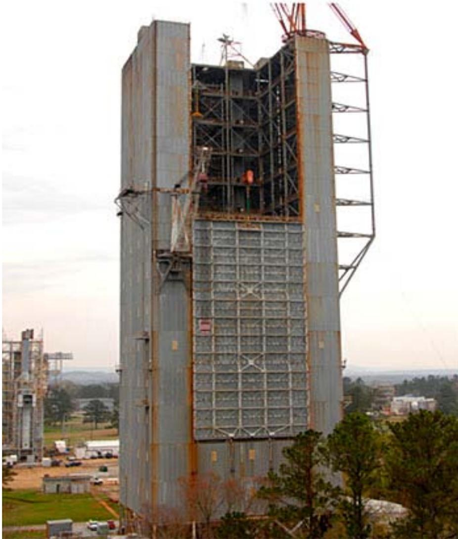
***In 2008, engineers and construction workers began refurbishing the Dynamic Test Stand at the Marshall Center for ground vibration testing of the Ares I.***
