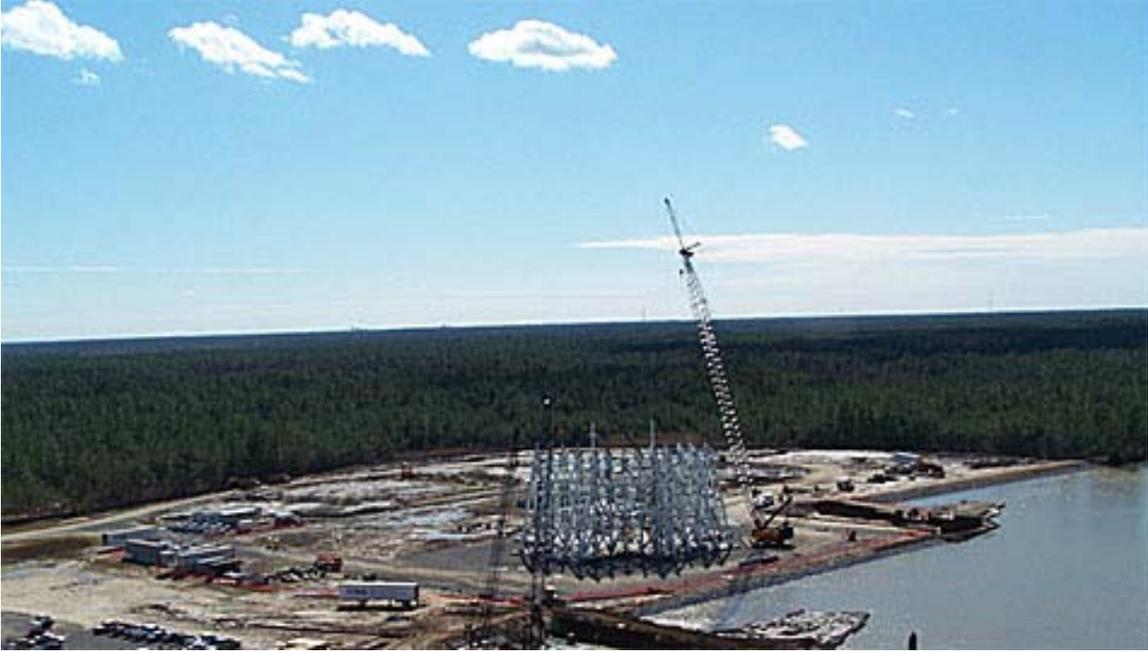
***For the first time in 30 years, NASA is building a new rocket engine test stand. In 2008, construction was started on the steel tower that makes up the A-3 test stand tower. The A-3 will be the first NASA stand capable of simulating atmospheric conditions similar to those the J-2X engine will experience when it is required to ignite and send the Ares I and Ares V into orbit.***
